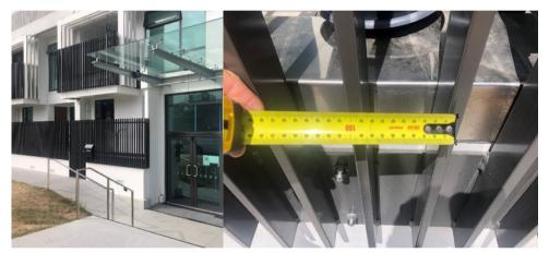
• Please confirm what is the general spacing between the metal fins of the railing. The desired outcome here is to provide only filtered views up from the pavement to the patios of the ground floor units while providing views out. This would suggest a narrower spacing for the fins of the railing.
